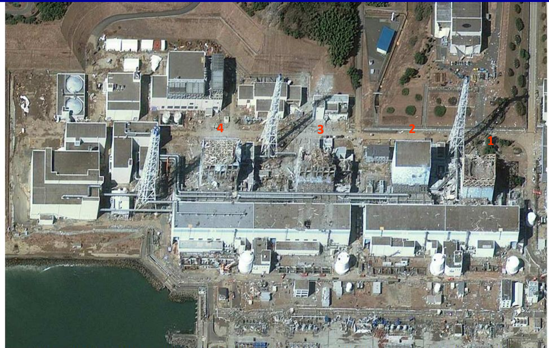
The damaged Fukushima Daiichi Power Plant in Fukushima is seen in this satellite image, taken and released on March 18, 2011. (Xinhua/AFP)
